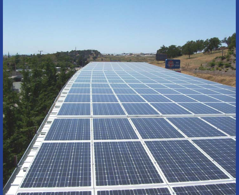
Jon's Pit Stop Construction Completed - Jackson
