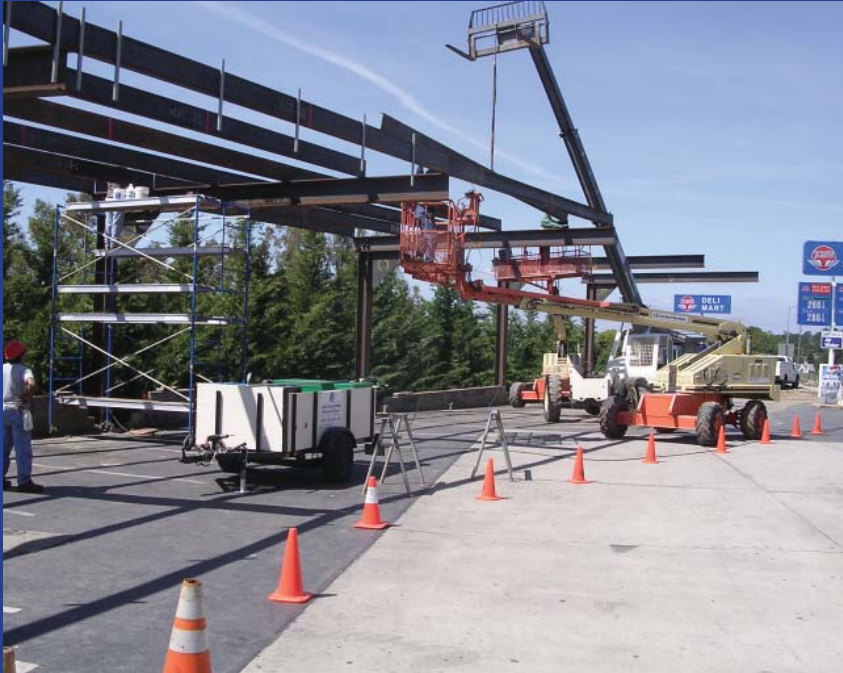
Jon's Pit Stop During Construction - Jackson
